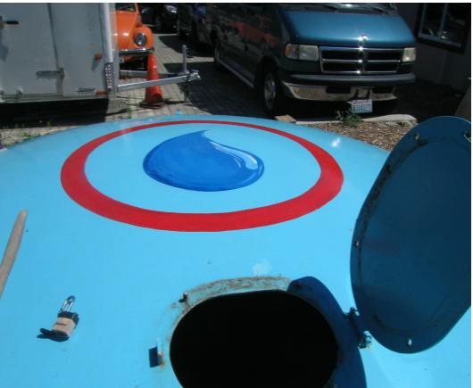
cistern top and access hatch
