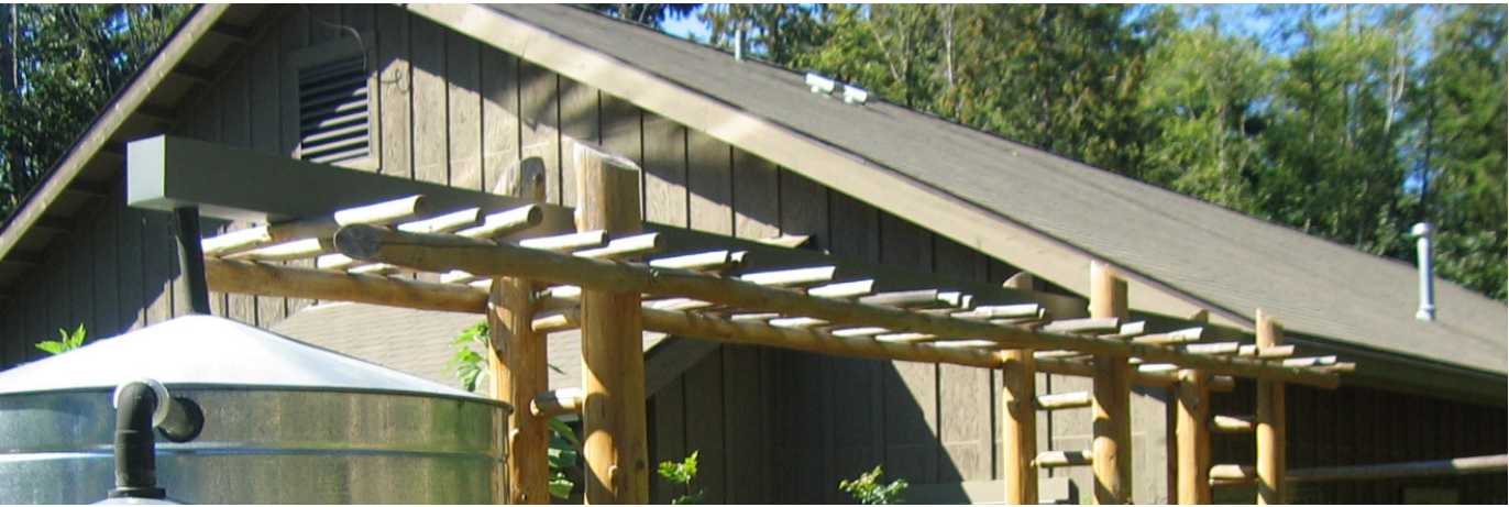
Islandwood rainwater conveyance system
