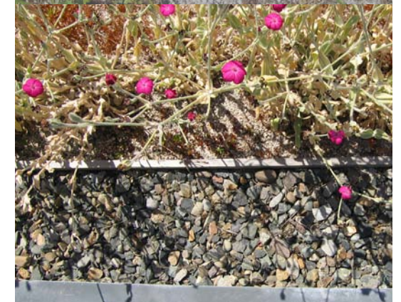
green roof edge condition
